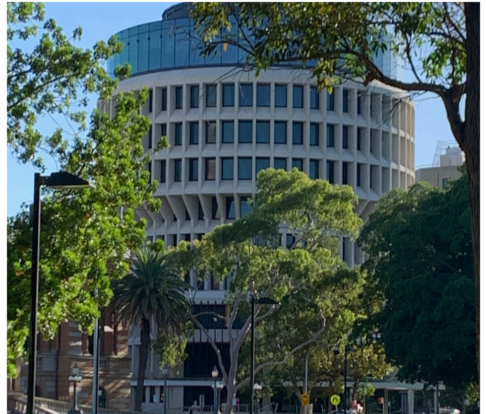
Former Newcastle Council Administration Building
