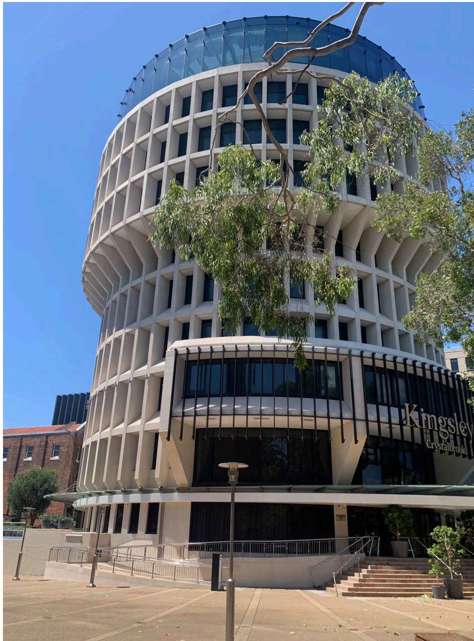
Former Newcastle Council Administration Building reinvented to become Crystalbrook Kingsley Hotel
