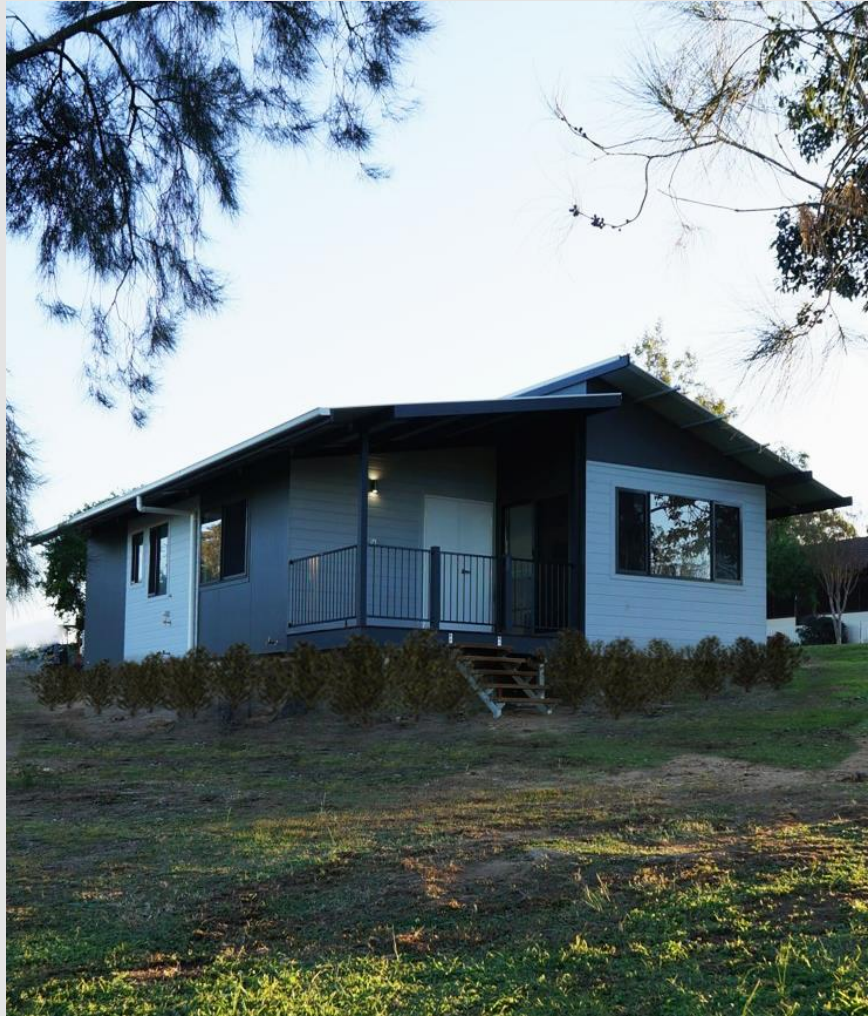
EXTERIOR VIEW OF FINISHED HOUSE ON SITE. YOURTOWN, NORTH RICHMOND
