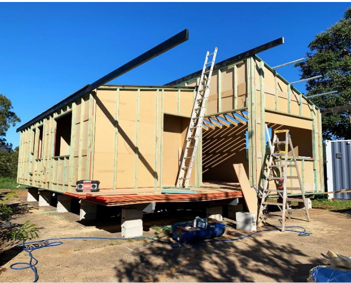
NEW COTTAGE BEING CONSTRUCTED OFF SITE GATEWAY CONSTRUCTIONS, CALOUNDRRA QUEENSLAND
