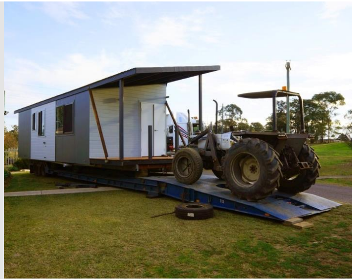
NEW COTTAGE BEING DELIVERED TO SITE YOURTOWN, NORTH RICHMOND
