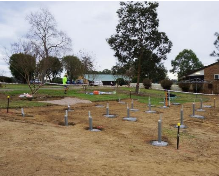
FOUNDATIONS ON SITE READY FOR COTTAGE DELIVERY YOURTOWN, NORTH RICHMOND
