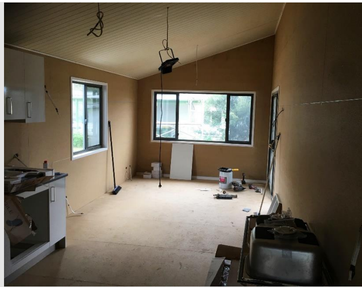
INSIDE COTTAGE DURING CONSTRUCTION OFF SITE GATEWAY CONSTRUCTIONS, CALOUNDRRA QUEENSLAND
